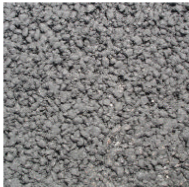
Figure 4.2: Bitumen coverage of aggregate at initial stage
