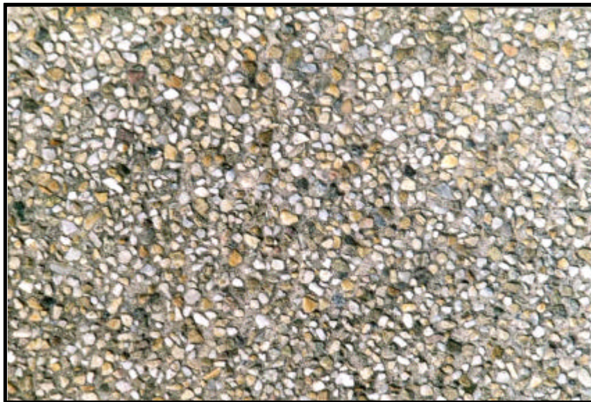
Figure 4.5: Example of an exposed aggregate cement concrete surface
