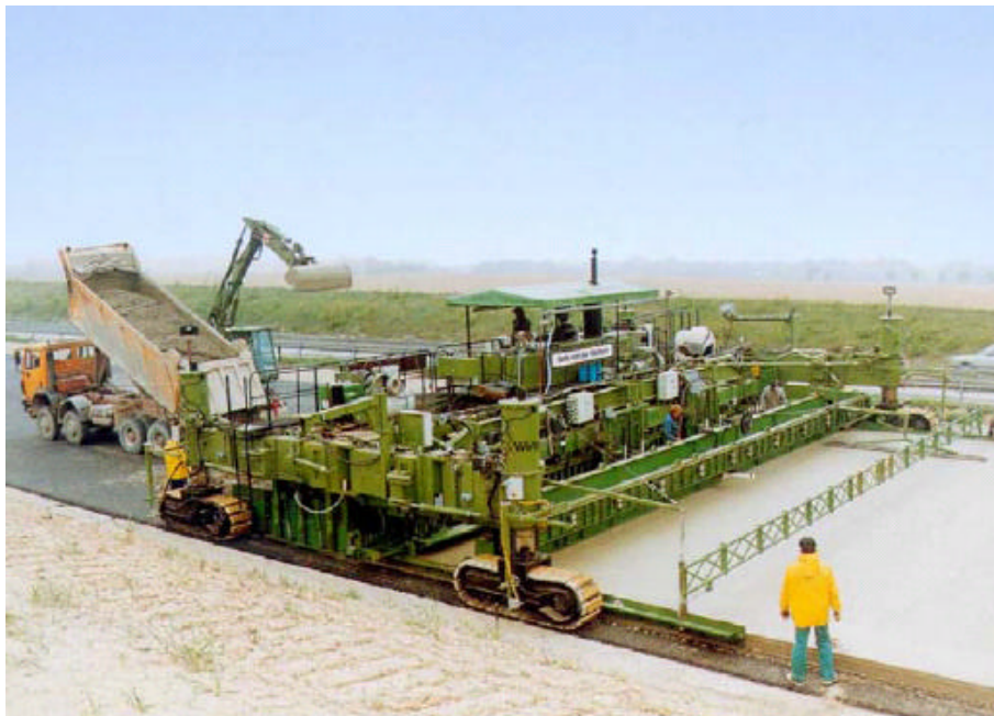
Figure 5.1: A slip-form paver in operation
